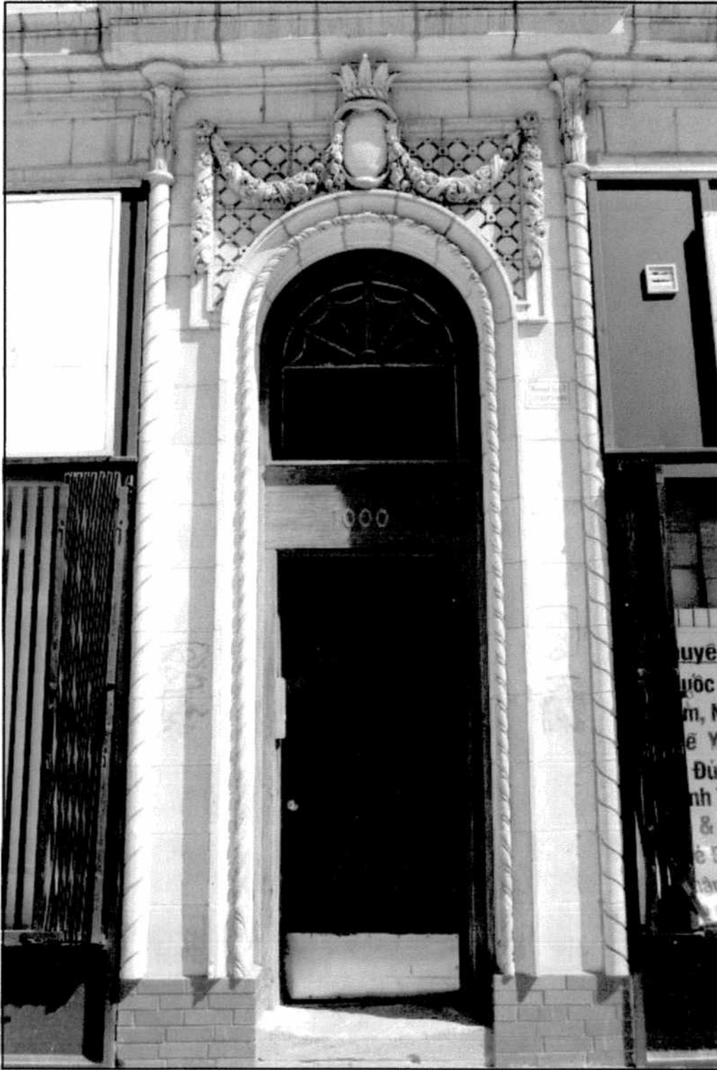
1000 West Argyle Street—Doorway detail
